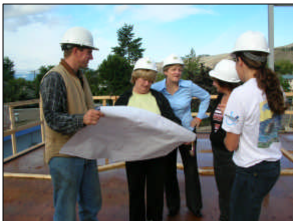
Shirley McGee goes over the plans with Bruce Young, Site Manager while atop the 2nd floor.
